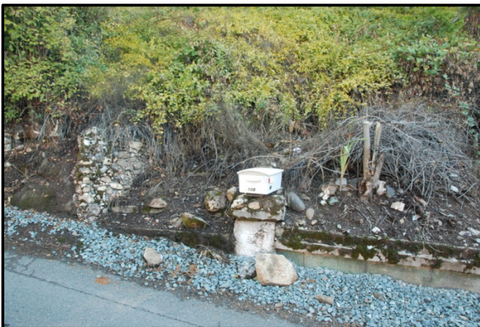
RESERVOIR STREET – LAYERED STONE RETAINING WALL (ON LEFT)
